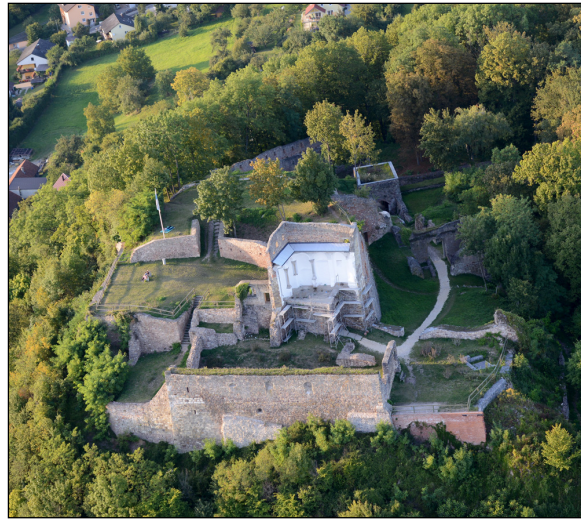
Figure 3: Aerial View of Donauauf Castle (Credit: ArcTron3D).
