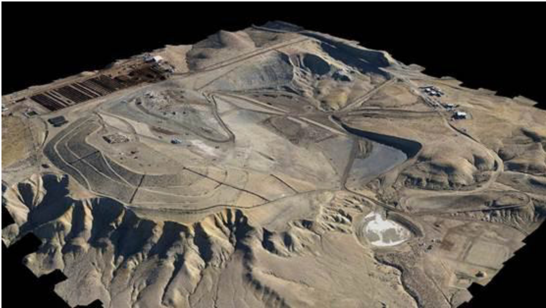
Figure 3: UAV data processing: DSM open pit mine with Trimble X-100 UAV data.
