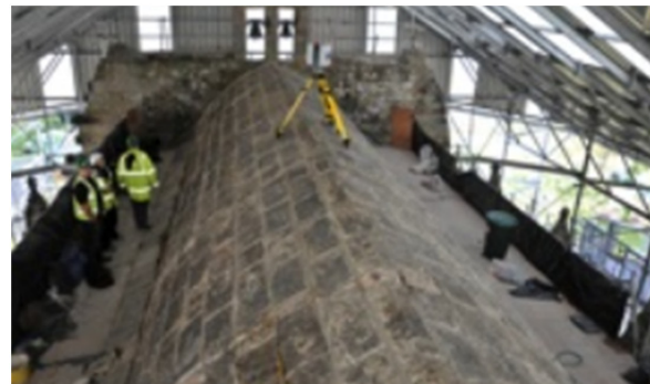
Image Two: Chapel vault with original exterior vault roofing removed and HDS6100 scanner in place
