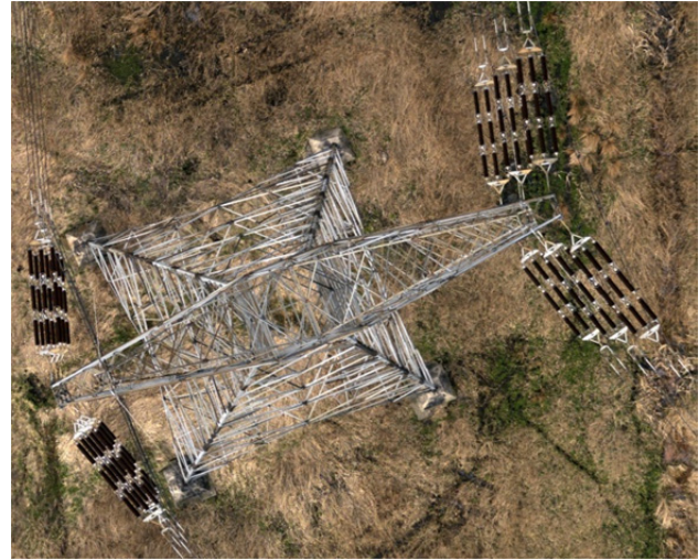
Figure 2: Power pole captured in nadir view.
