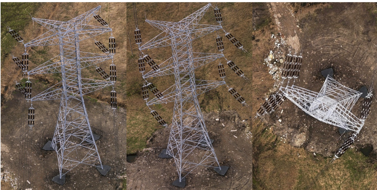
Figure 9: Point cloud and photo of the same pole for the forward, backward and nadir view.
