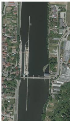
Figure 17: True Orthophoto (DOP) of the lock Hessigheim.
