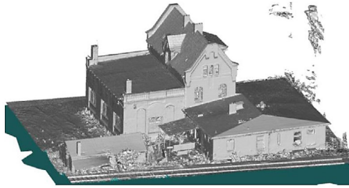
Figure 14: Meshed surface of the building, generated from UAV images. A precise, homogeneous and complete reconstruction was achieved with the well-distributed images of our flight planning and execution concept.
