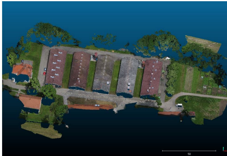
Figure 15: Dense point cloud of visible surface derived from SURE software. The farm buildings are completed modeled, parts of vegetation can also be seen.
