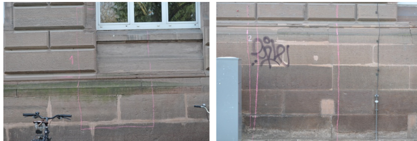
Fig. 9: Two areas on the façade (Area 1: left, Area 2: right)
