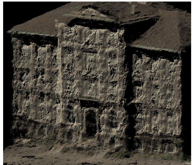
Fig. 6. Facade image in oblique view and corresponding 3D point from dense image matching.
