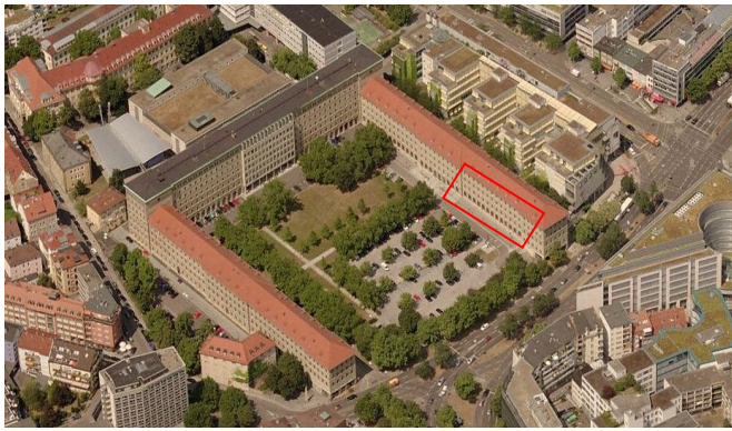
Figure 1. Birdseye view on the “Rotebühlbau, Stuttgart” (source: Bing Maps). Red rectangle marks the façade part for which images were collected and 3D reconstruction was performed.
