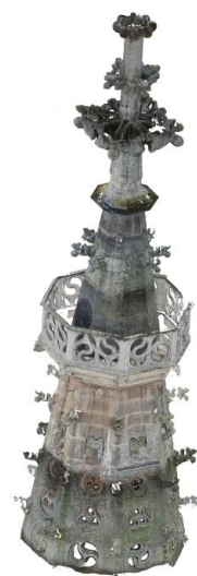
Figure 5: The six point clouds captured from the scaffold registered into a common coordinate system.
