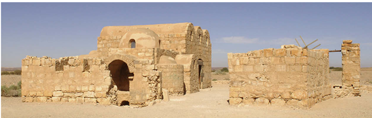
Fig. 2. Serious longitudinal cracks extended through the Amra palace walls (World Cultural Heritage Site).
